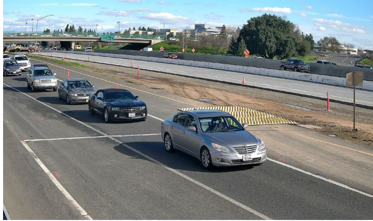
Figure 14: Reduction of the On-Ramp from Three Traffic Lanes to One Traffic Lane.
