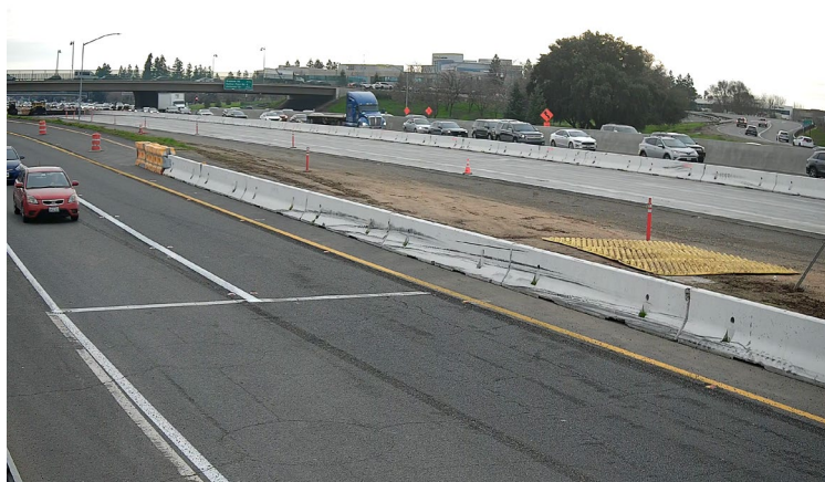
Figure 15: Reconfigured Roadway with Two Traffic Lanes and One Merging Lane.
