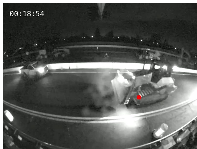
Figure 17: Construction Activity on the On-Ramp.
