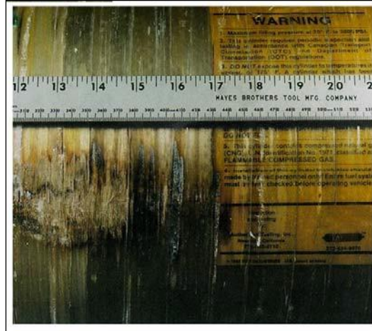
Figure 11-20. Level 3 Heat Damage to a Type 4 Container
