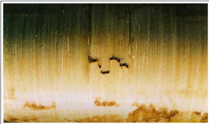
Figure 11-17a. Level 3 Stress Corrosion Cracking and Chemical Damage to Container
